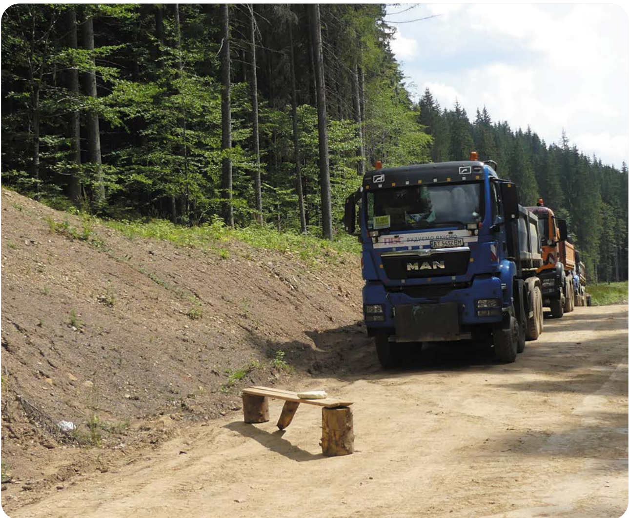
New “forest highway” under construction of PBS LLC, August 2023
